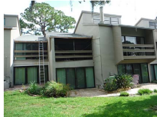
4 Left Side of Building C
