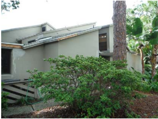
3 Rear of Building C
