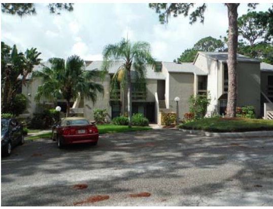
1 Front of Building C
